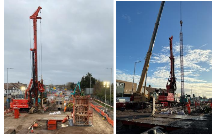
Images 1 and 2: piling operation
