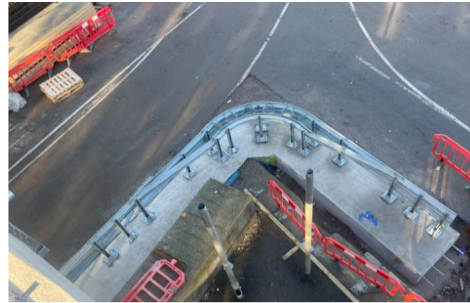
Image 4: Roadside crash barriers on A127
