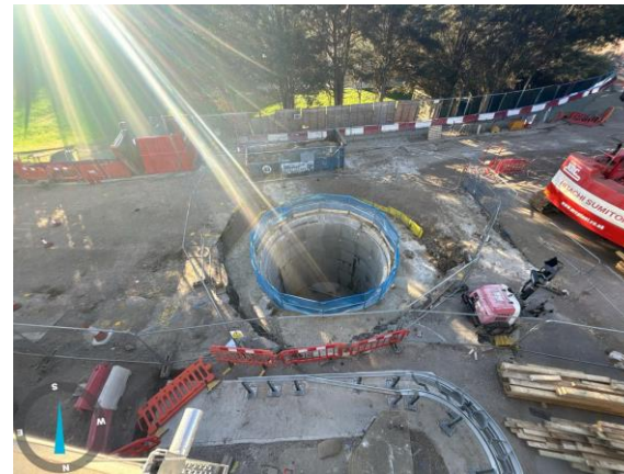
Image 7: The new reception pit to enable tunnelling work
